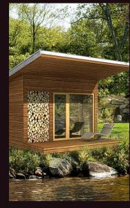
The PUUTALO 1 type is realized as a timber building, based on the concrete piles. The building is designed in a "two-by-four" system, from beams with the cross-section of  $120 \times 60$  mm. There is a shed roof with an overhang.
